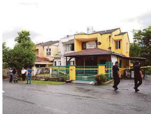
The affected occupants in Jalan Kelab Ukay 4 are allowed only to take their belongings and will not be allowed to live in their homes for the next six months. PIC BY FATHIL ASRI
